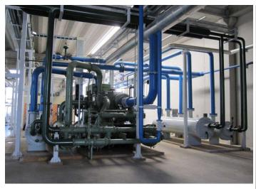
The 5L Series is a modular, "packaged" type plant furnished in eight modules: feed air compressor, recycle air compressor, air chiller, pre-purifier, turboexpander and three cold boxes. Two standard models are available with production capacities of 3000 and 5000 Nm<sup>3</sup>/hr.
