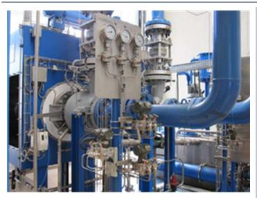
The 4L1000 is a modular, "packaged" type plant furnished in six modules: feed air compressor, recycle air compressor, air chiller, pre-purifier, turboexpander and cold box.
