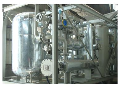
The 3L500 is a modular, "packaged" type plant furnished in six modules: feed air compressor, recycle air compressor, air chiller, pre-purifier, turboexpander and cold box.
