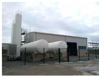
The 2L300 is a modular, air-cooled, "packaged" type plant furnished in five pre-assembled modules: dual feed air compressors, air chiller, pre-purifier and cold box. The dual – warm and cold – turboexpander system provides highest plant efficiency available in this plant size range
